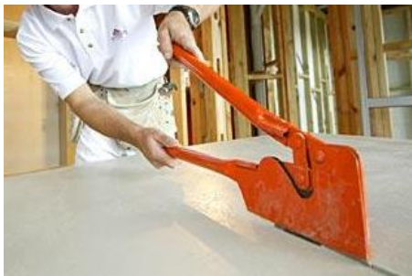
Cutting fibre cement sheets
